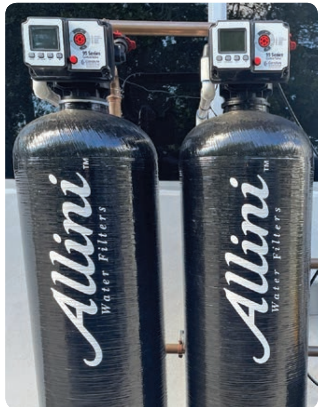
PHOTO PROVIDED BY MARINE INDUSTRIES ASSOCIATION OF SOUTH FLORIDA
